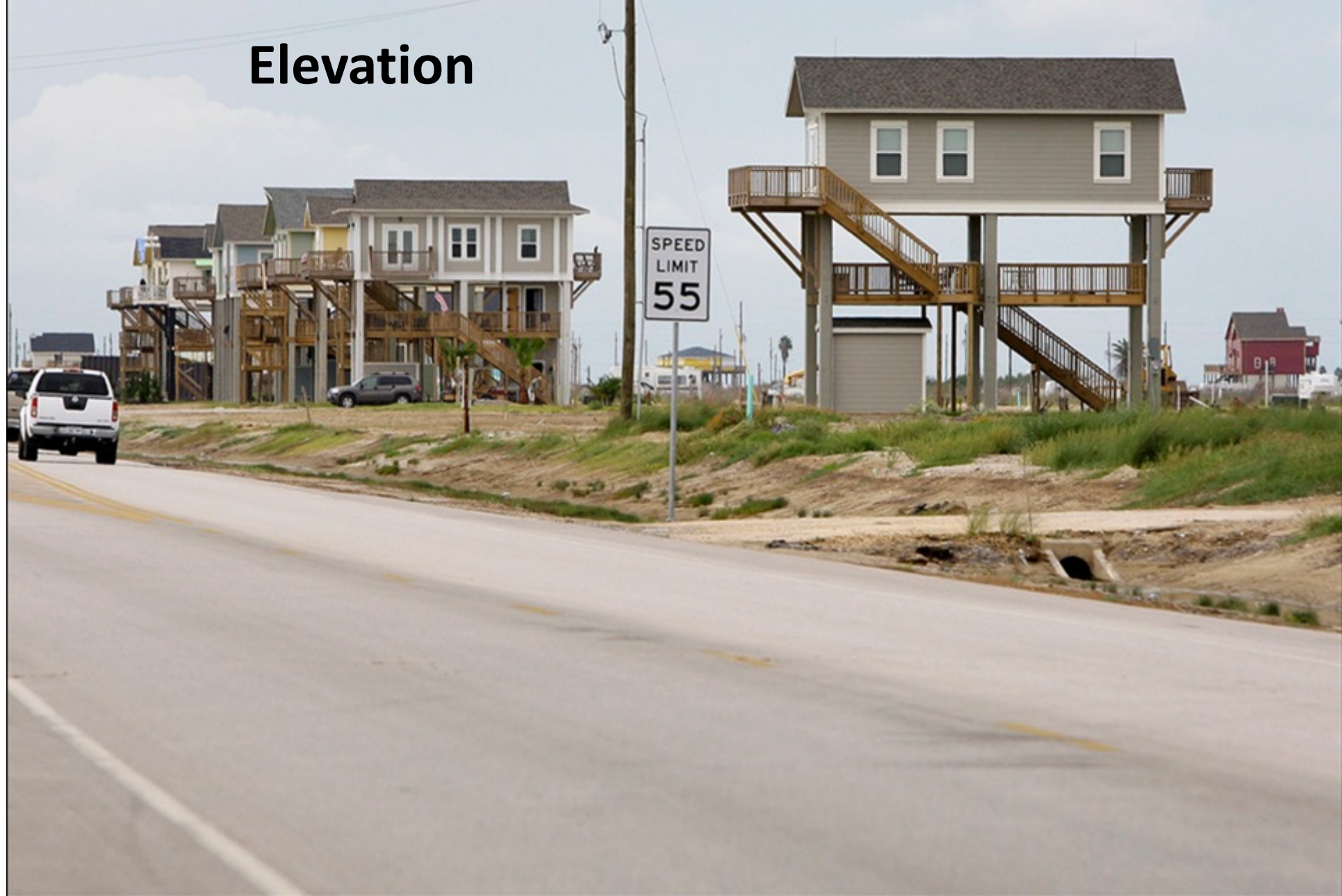
8 A pair of photos showing what locals refer to as the "Bird Houses", because of the building design, near Gilchrist Texas. The first photo was made Sept. 16, 2008, showing where Hurricane Ike's surge had washed sand and debris over Highway 87. The second photo was taken on Sept. 9, 2009. [click image to see it fade] (AP Photo/Tony Gutierrez)#
